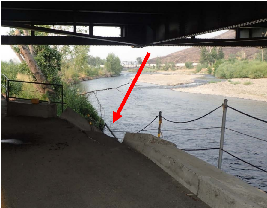
Photo 2. Damage located under the bridge includes erosion along the toe and undermining of the trail so that it is falling into the river. Photo is taken looking upstream along the Naches River from under I-82.
