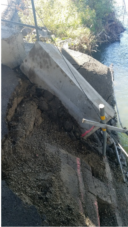
Photo 3. Another view of the damage underneath the bridge showing material eroding into the river below the bridge.
