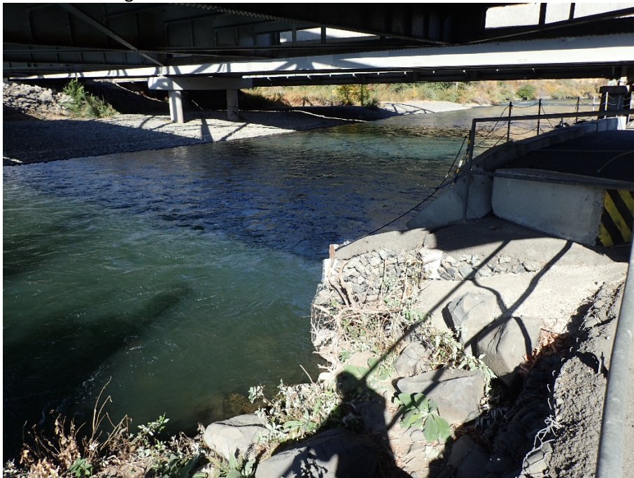
Photo 4. Another view of the damage underneath the bridge, including armor and exposed gabion boxes and concrete bridge foundation.
