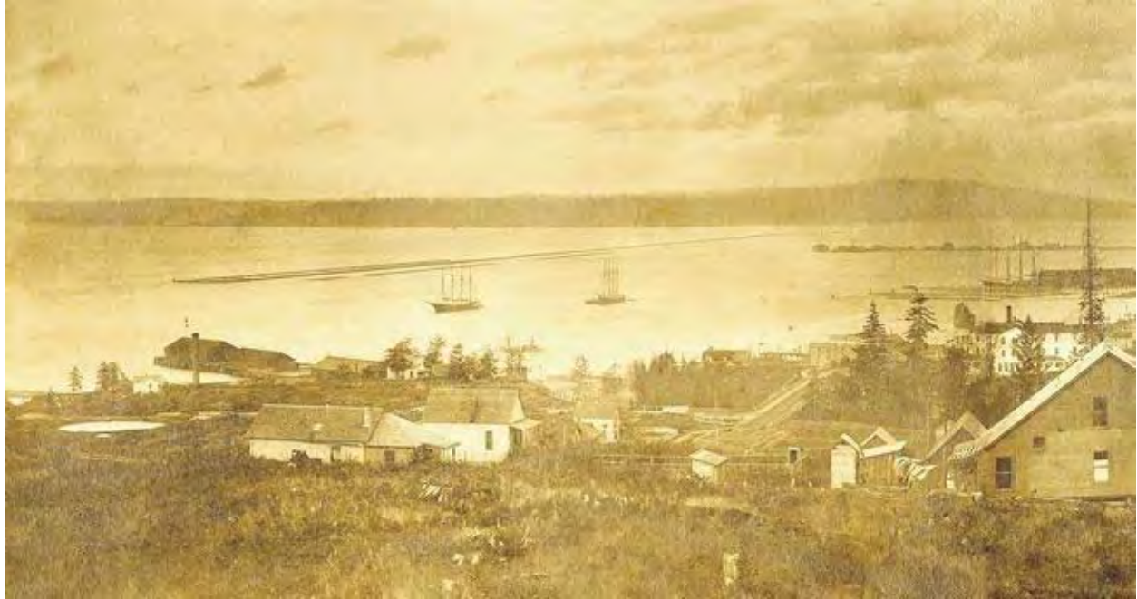
Figure 21. Everett waterfront in 1902 showing the jetty before it was buried with dredge material creating Jetty Island, which protects the exposed waterfront.
