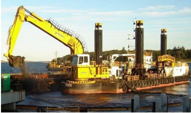
Figure 4. Excavator dredge with a hydraulic arm and scoop bucket on a spud barge.
