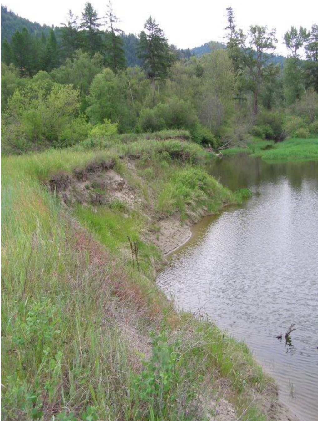
Photo 4: Dunn Creek Bank Stabilization site
