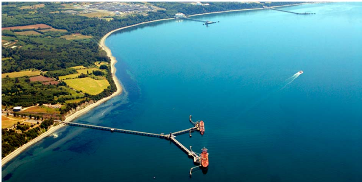
Figure 1. BP Cherry Point Facility Docks
