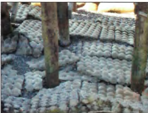
PHOTO 4: EXISTING CONCRETE REVETMENT
