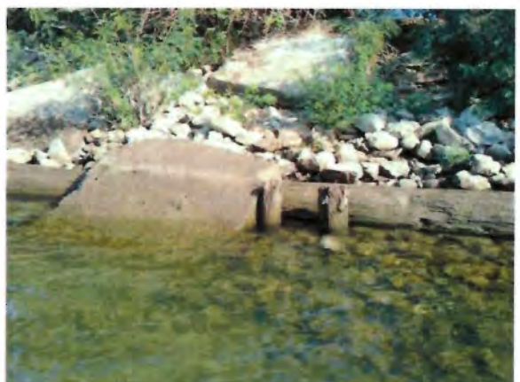
Photograph of concrete riprap along bank facing North
