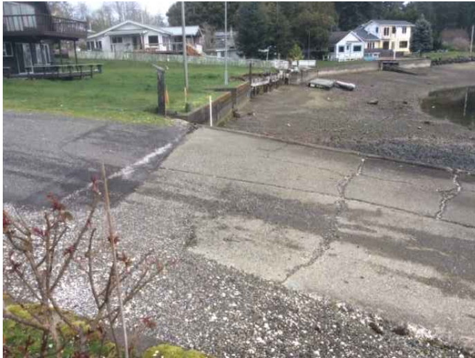
PRE-EXISTING CONDITIONS - PROJECT SITE LOOKING NORTH AT DOCK LANDING
