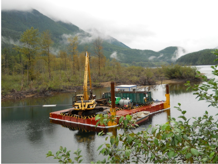
Figure 7. An example of a floating pad using Flexifloat.
