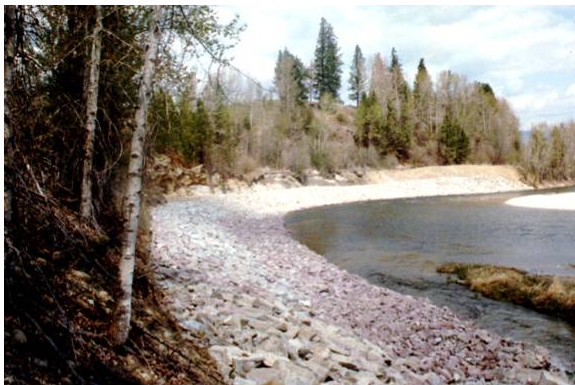
Figure 2.25 ACCEPTABLE riprap for erosion control. (MT)
