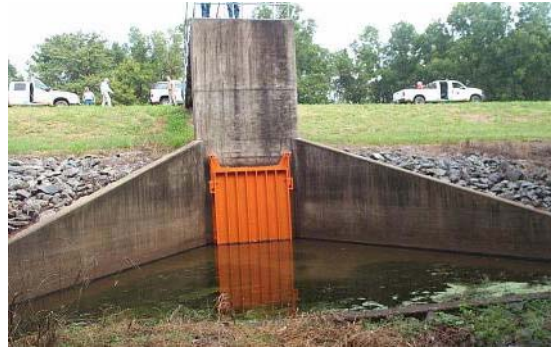
Figure 2.63 ACCEPTABLE culvert gate. (LA)
