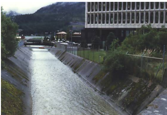
Figure 2.74 ACCEPTABLE concrete lined channel. (AK)
