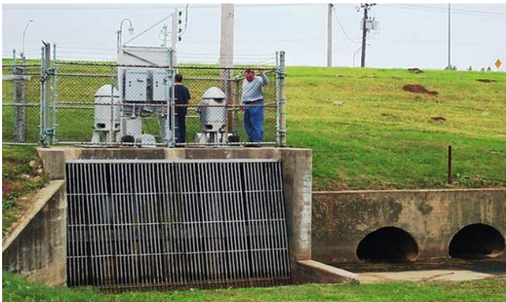
Figure 2.68 Pump station beside earthen levee. (OK)
