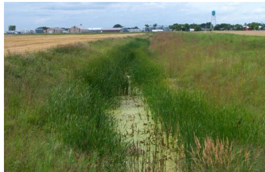
Figure 2.55 MINIMALLY ACCEPTABLE vegetation (cat tails and bull rushes) in interior drainage ditch. (MN)
