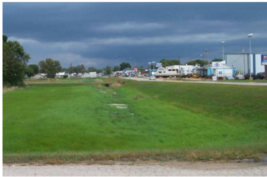
Figure 2.54 ACCEPTABLE interior drainage channel. (IA)
