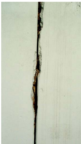
Figure 2.45 UNACCEPTABLE exposed rebar. Monolith joint separation with exterior spalling along the joint and interior spalling in the area of the rebar. (MN)
