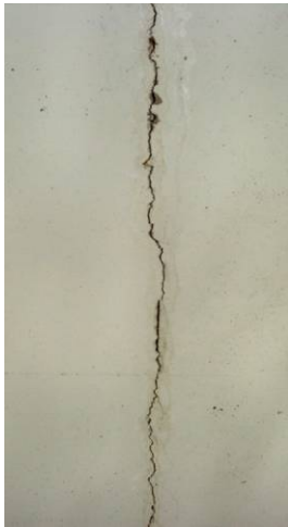
Figure 2.43 MINIMALLY ACCEPTABLE 1/8 th inch crack extends through concrete floodwall and needs to be sealed to prevent further damage. (MN)
