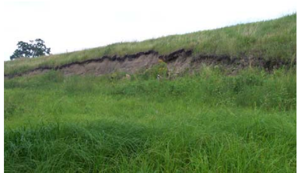
Figure 2.17 UNACCEPTABLE earthen embankment failure. (MN)
