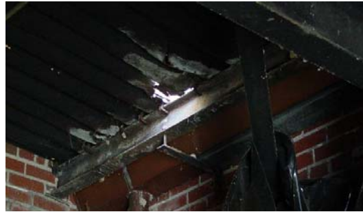
Figure 2.67 Hole in roof of pumping station. (IL)
