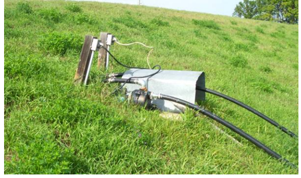
Figure 2.8 UNACCEPTABLE encroachment. Piping for lawn irrigation system drilled through levee without approval. (ND)
