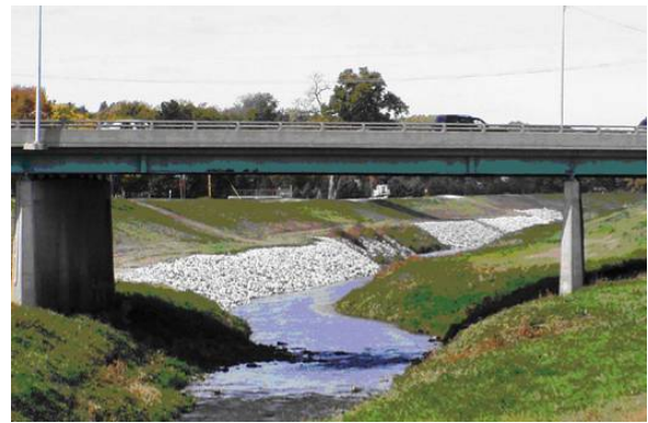
Figure 2.26 ACCEPTABLE riprap for erosion control. (NE)
