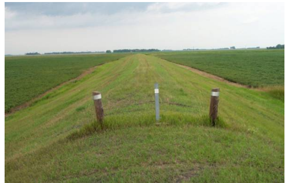
Figure 2.5 MINIMALLY ACCEPTABLE. Field encroaches on levee easement. The landowner has tilled the soil right to toe of the levee, and was requested to stay back at least 10 feet. (ND)
