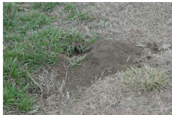
Figure 2.20 Animal burrow in a levee. (IA)
