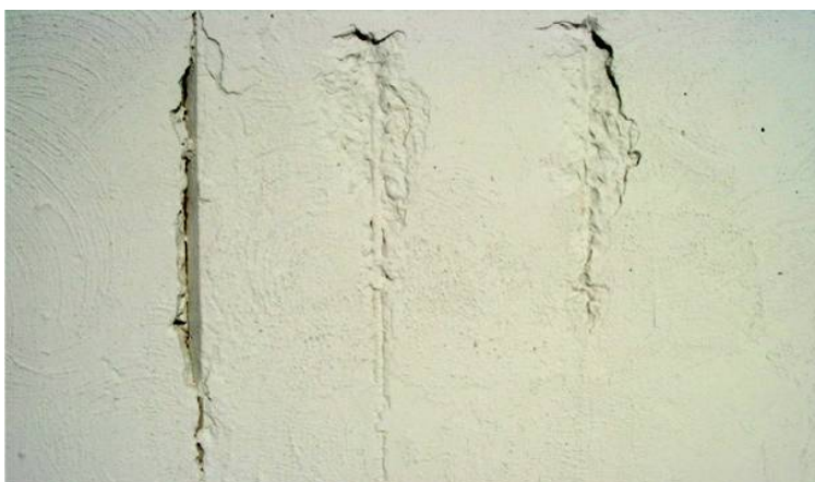
Figure 2.47 MINIMALLY ACCEPTABLE floodwall. Exposed surface rebar resulting from poor construction practices. The public sponsor has painted over the rebar in an attempt to keep it from rusting. (MN)
