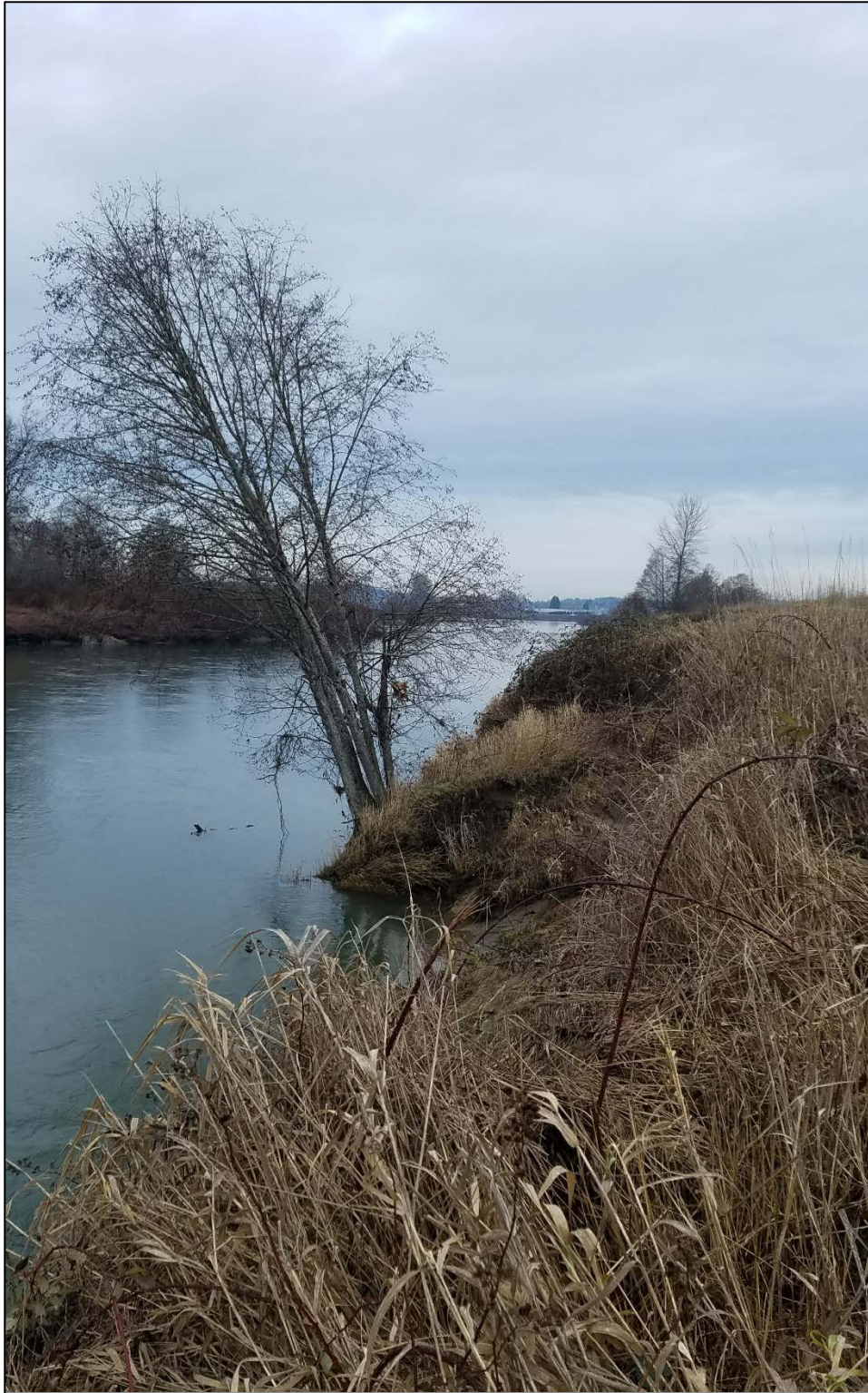
Figure 5. Red alder within slumped material at damage site (photo taken Jan 2018).
