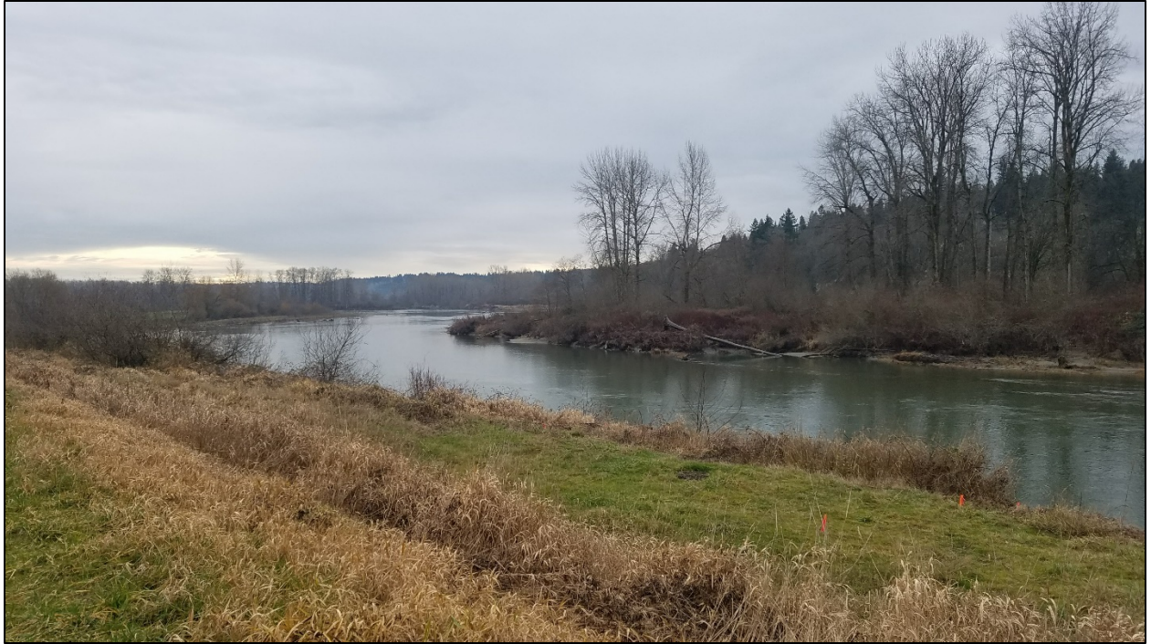
Photo 2. Lord Hill site looking upstream from the damaged location.
