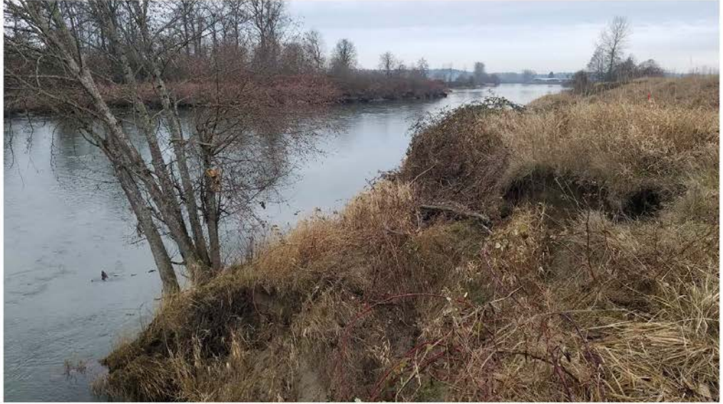
Figure 5. Red alder within slumped material at damage site (photo taken Jan 2018).
