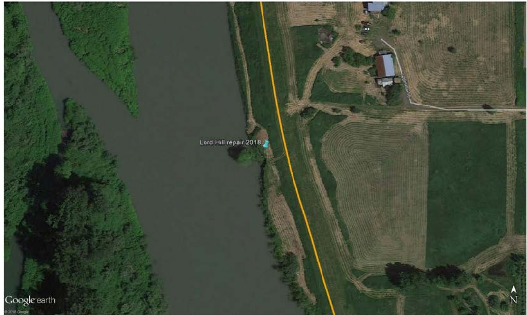
Figure 2. View of the levee repair location and tree caught within slumped material.
