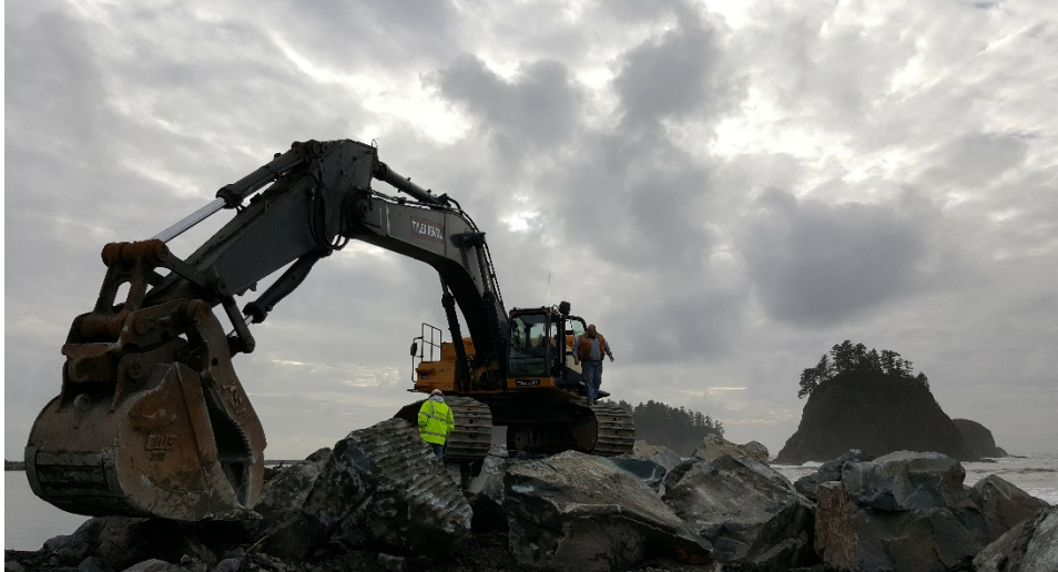
Figure 3. Examples of typical repair activities: working along the road (top), bringing out individual rocks due to their large size (middle), and positioning rocks by excavator (bottom).
