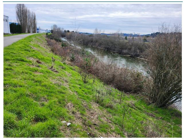
Photo A-2 Desimone levee at approximately RM 15, upstream orientation. Grass and small, dispersed vegetation on riverward slope. Instream LWM on opposite riverbank established in 2008 repair. February 2024.
