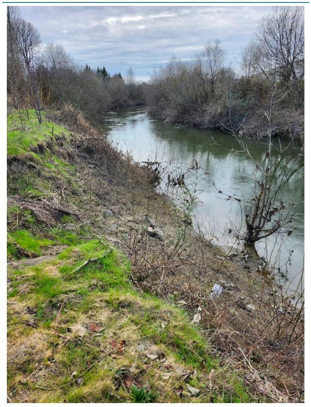
Photo A-5. Erosion of riverward levee face. Scattered riprap over mixed earth. Upstream orientation. Approximately RM 15.15.
