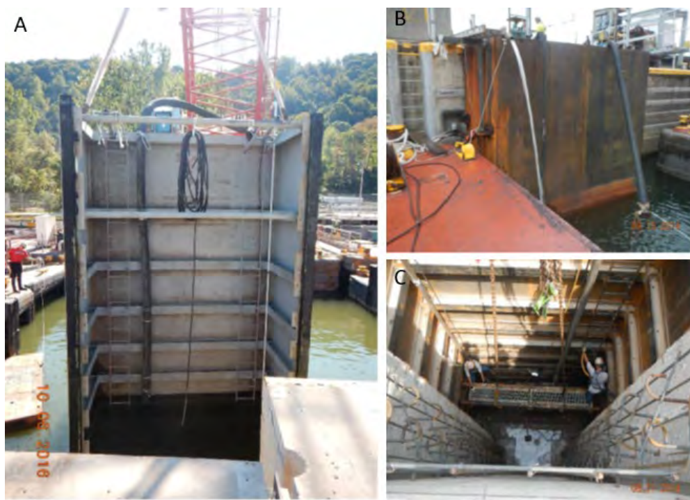
Figure 5. (A) Localized cofferdam example. (B) Example of an installed localized cofferdam. (C) Example of the inside of a localized cofferdam.
