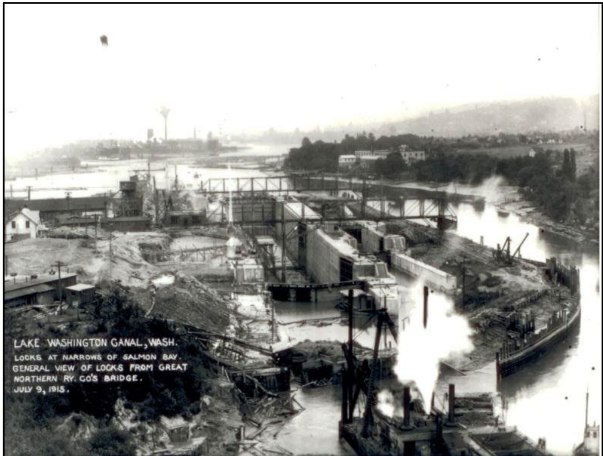
Figure 2. Construction of the Locks, looking east, 1915, prior to development of the circulation system and terraced lawn.
