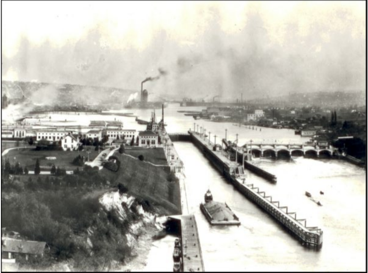
Figure 8. View of the Locks and grounds (left) looking east from the Great Northern Railroad Bridge, post 1916.
