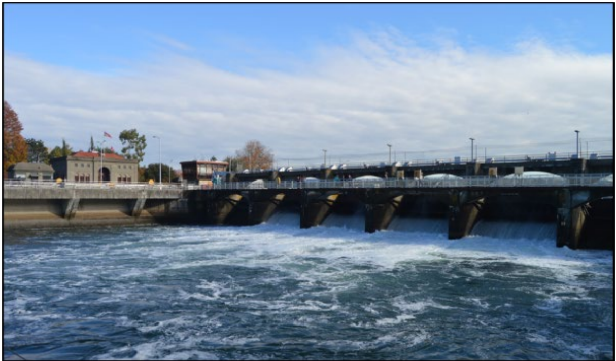
Figure 6. The Locks dam and spillway gates in October 2016.
