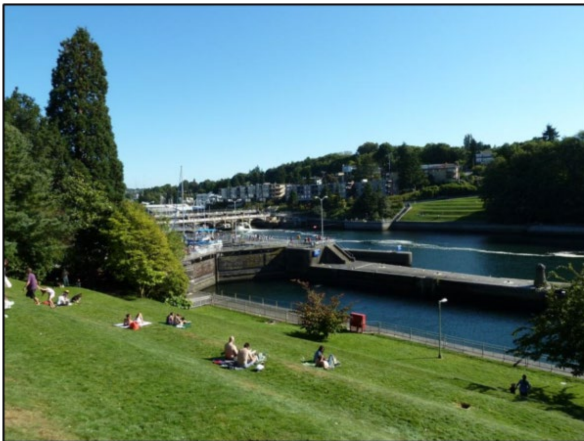
Figure 19. View looking southeast of the terraces from the overlook toward the Locks and dam (Photograph courtesy of the National Park Service, Pacific West Region 2012).
