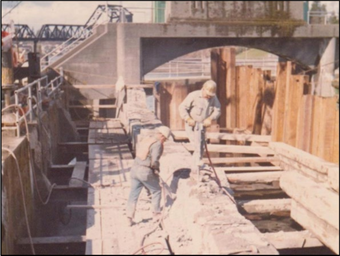
Figure 7. Renovation of the fish ladder in 1976.
