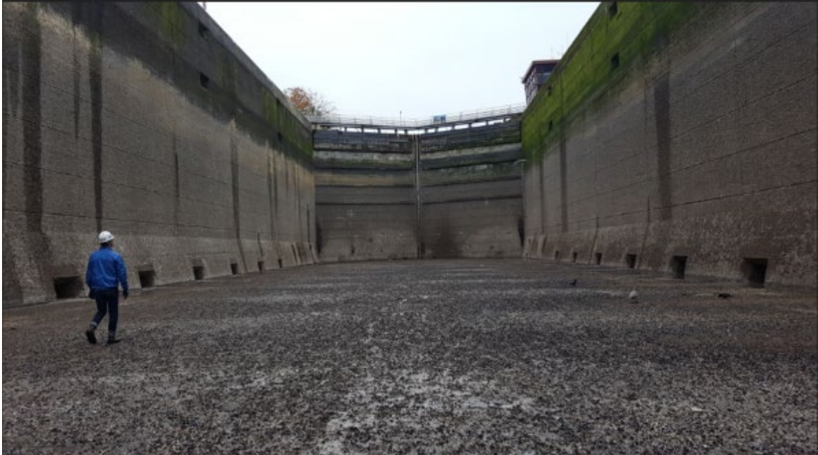
Figure 27. Large lock dewatered in preparation for maintenance work in 2019.
