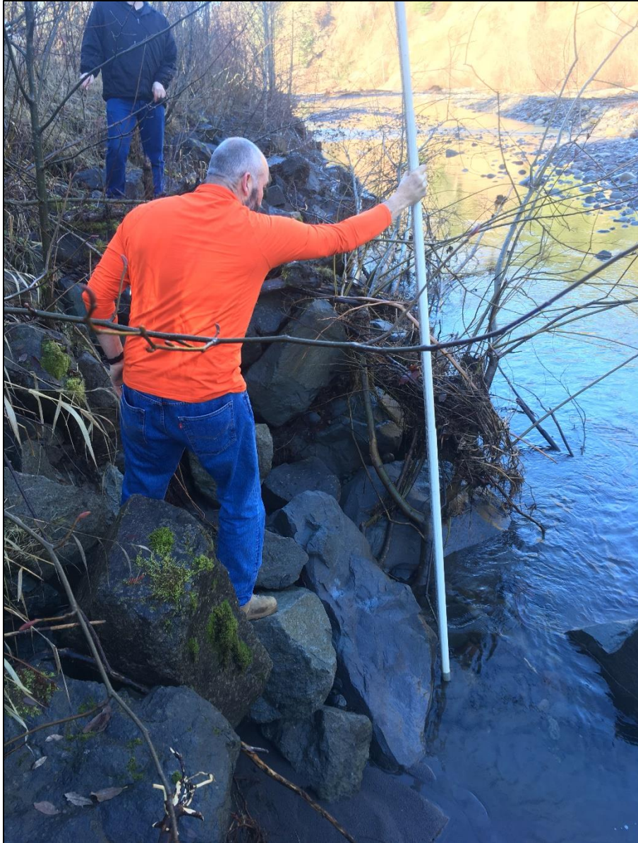
Photo 3. Alward 1 Site 3, missing riprap and damage to the slope and toe.
