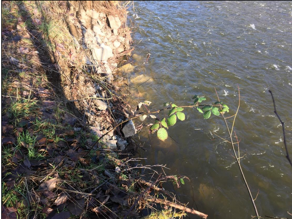
Photo 4. Bridge Street Site 1, looking downstream the levee slope is a certical face at the waterline.
