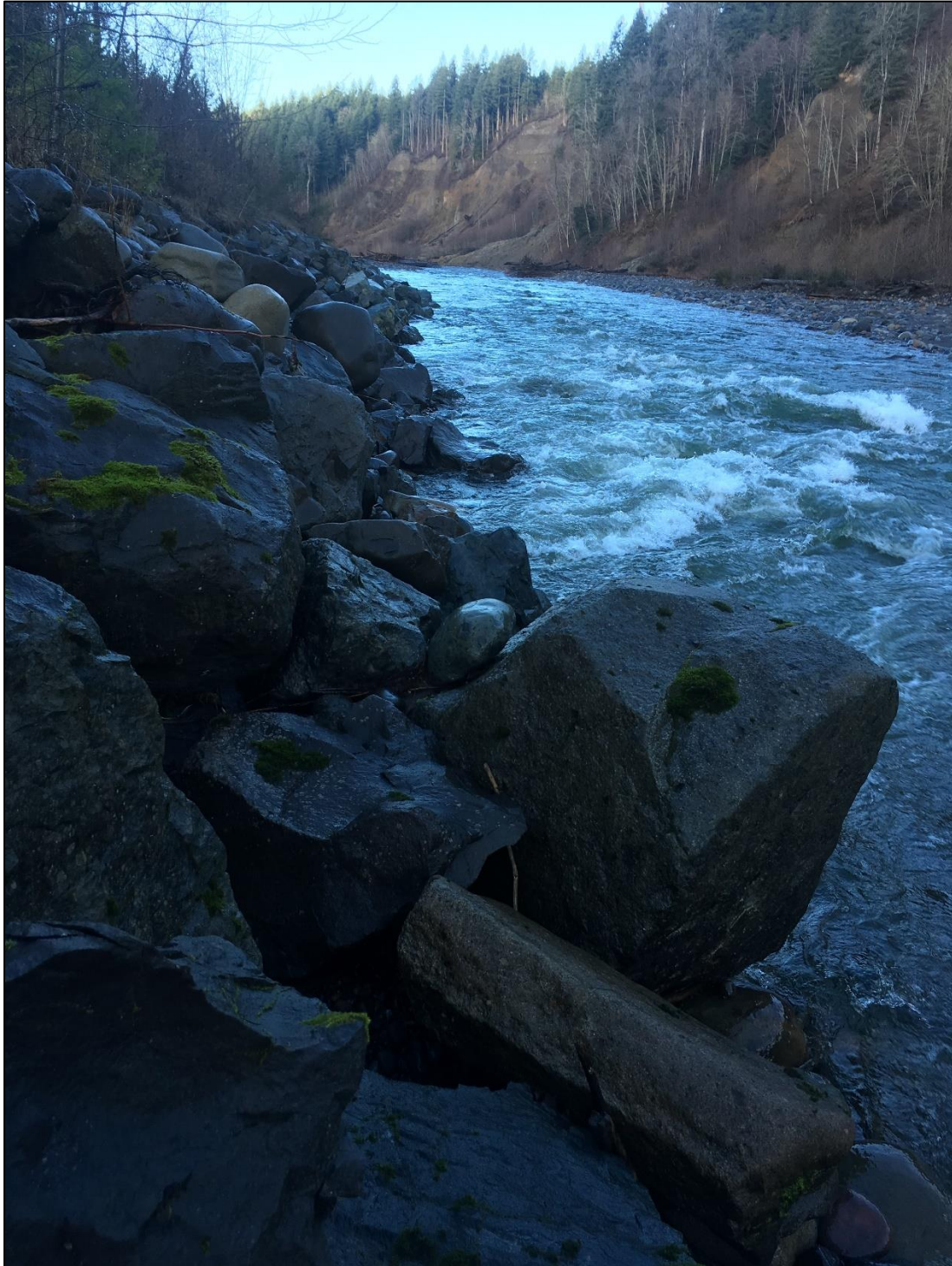
Photo 1. Alward 1 Site 1, damage to the lower slope and toe.
