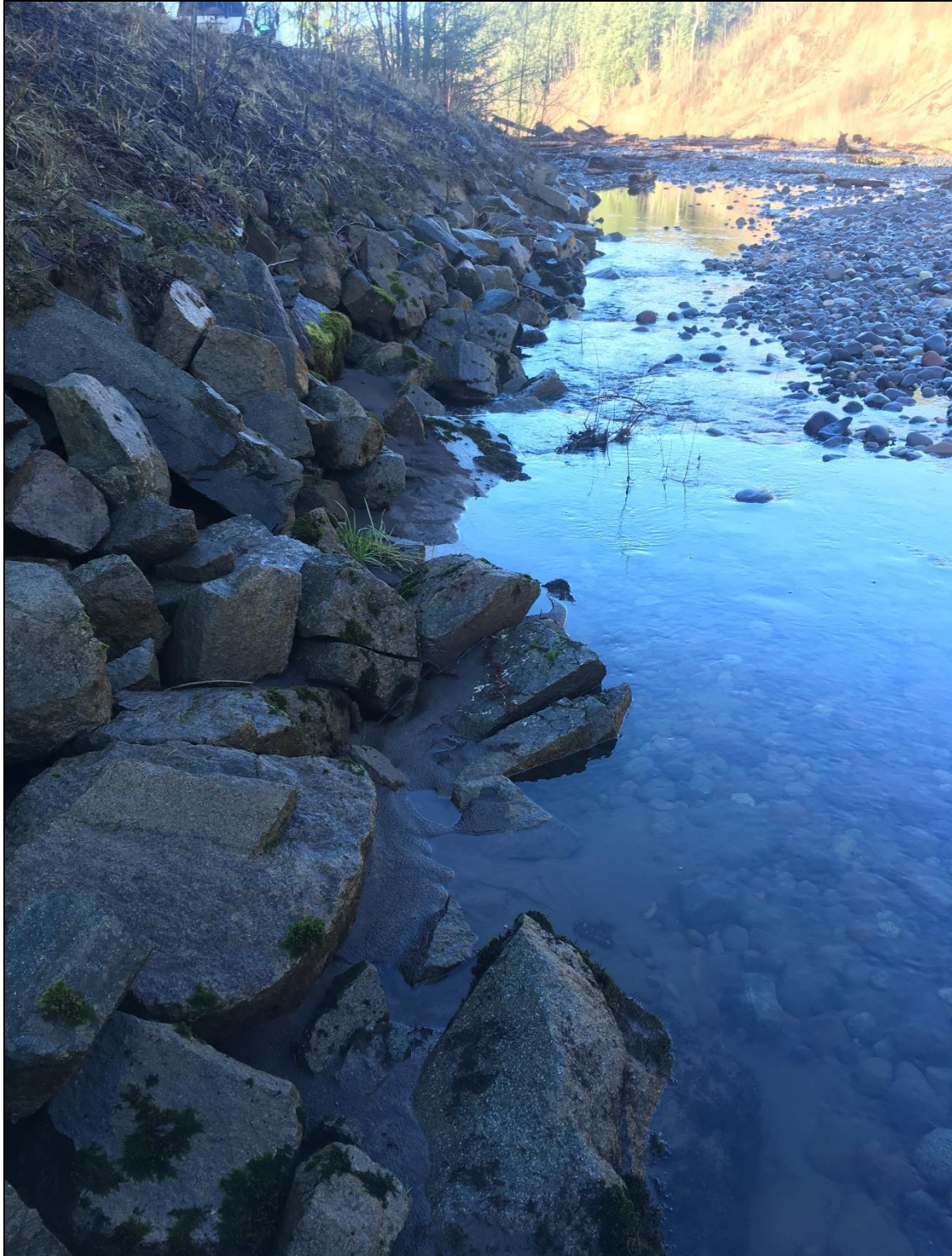
Photo 2. Alward 1 Site 2, missing riprap and damage to the lower slope and toe.
