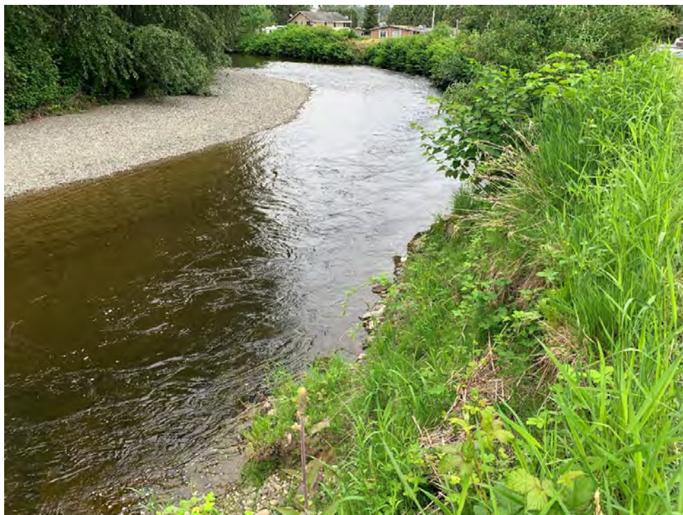
Photo A1. Bank caving and erosion at Pilchuck Levee toe looking upstream.
