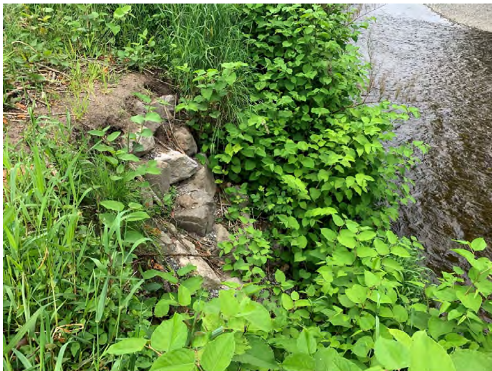
Photo A3. Erosion and temporary repair at the Pilchuck Levee looking downstream.
