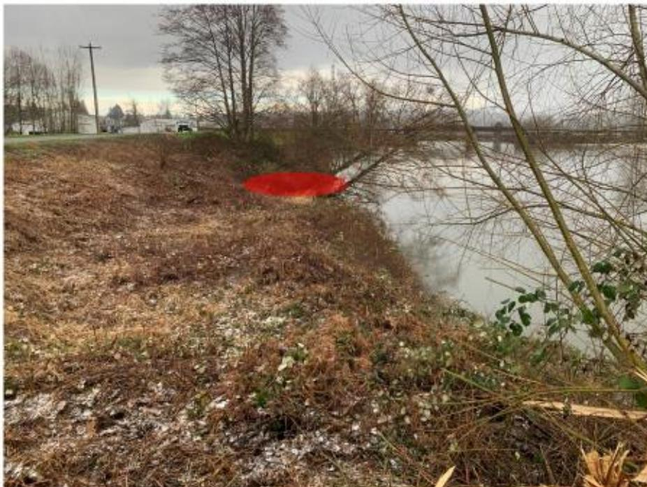
**Photo 2:** Scour hole, shown in red, on the riverward slope, downstream oriented (198+00).
