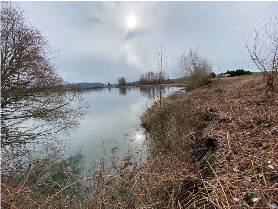
**Photo 4:** Scour hole and subsequent sloughing on the riverward slope, upstream oriented (STA 199+50).
