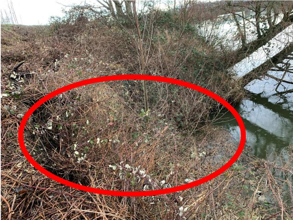
**Photo 1:** Riverbank Erosion, shown in red, downstream oriented (197+50).
