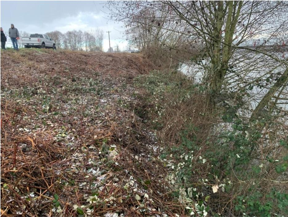
**Photo 3:** Sloughing landward of the trees on the riverward slope, downstream oriented (199+50).
