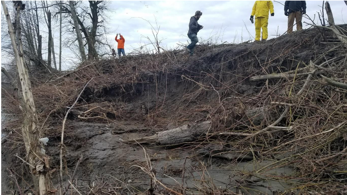
Photo 3: Embankment scour at Site 1 located within the middle of the damaged length.
