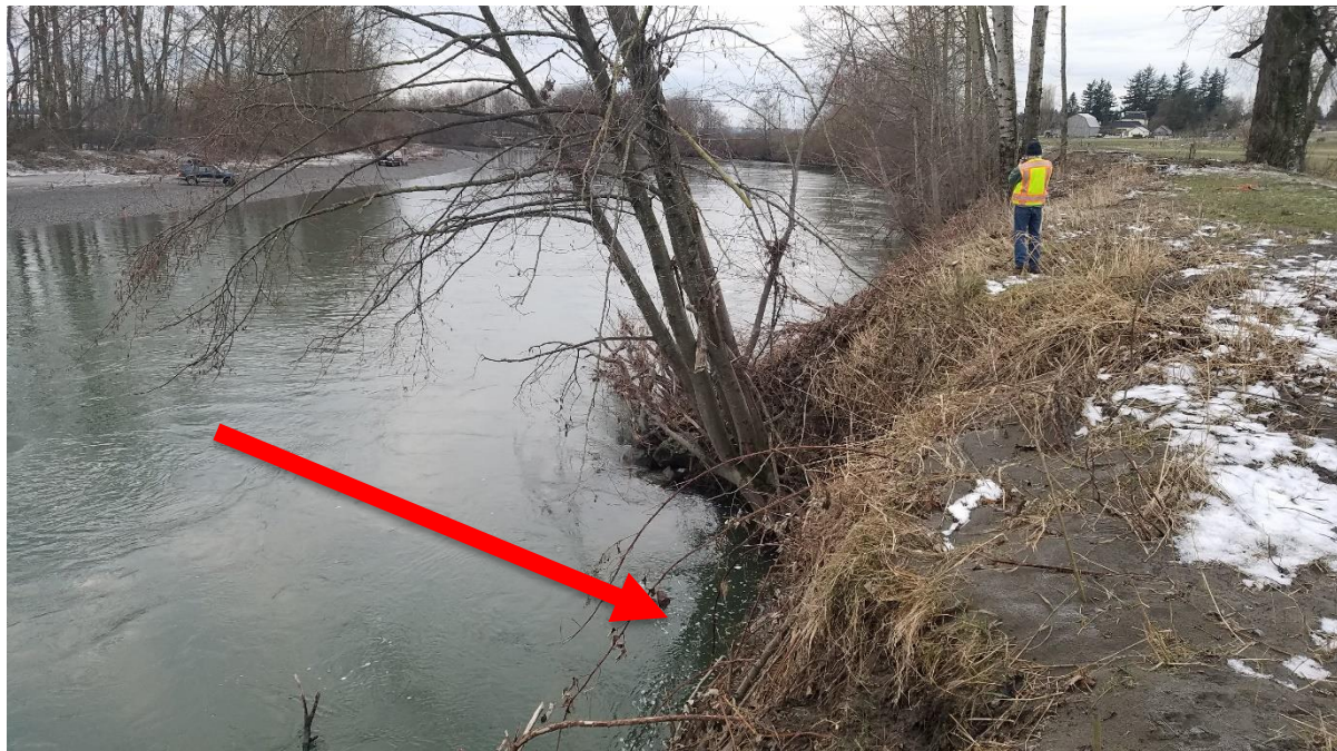
Photo 2: Toe scour into levee prism at the downstream end of Site 1
