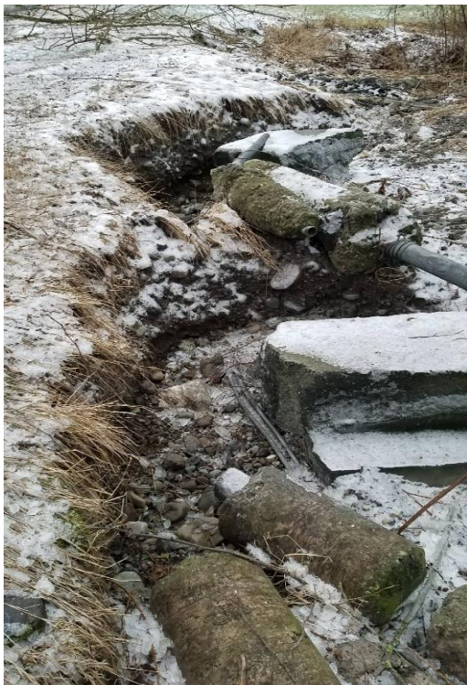
Photo 6: Overtopping damage on the landward crest at Site 1.
