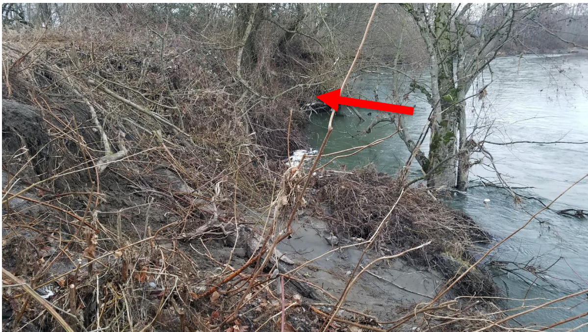
Photo 4: Looking upstream from embankment scour shown in photo 3. Arrow points to where the perched outlet from culvert drainage enters into the Nooksack River.
