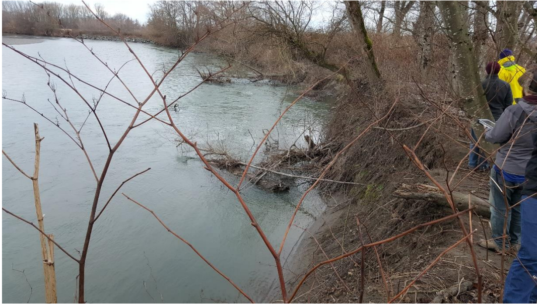
Photo 7: Toe scour into levee prism at Site 2.
