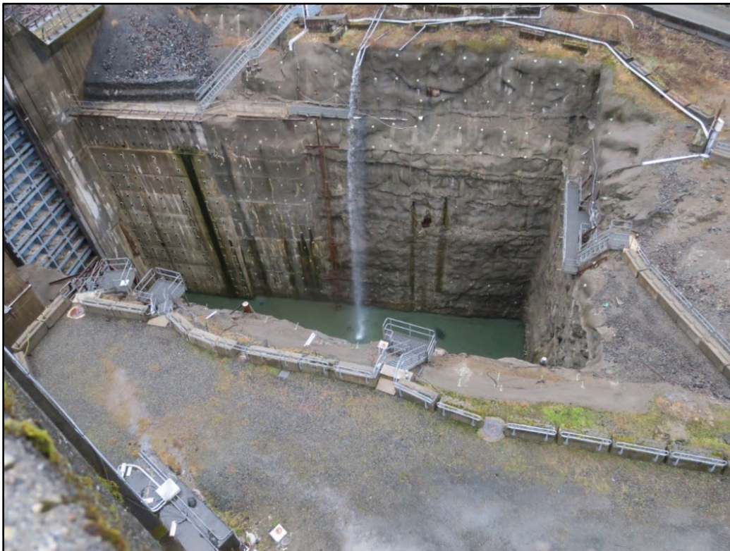
Figure 1-3. Fish passage facility excavation.
