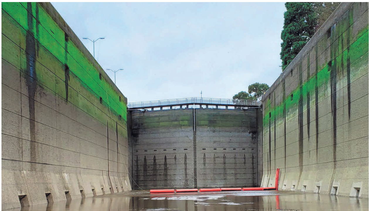
Enclosure 5. De-watered, double skin, historic center gates, photo taken March 2021.
