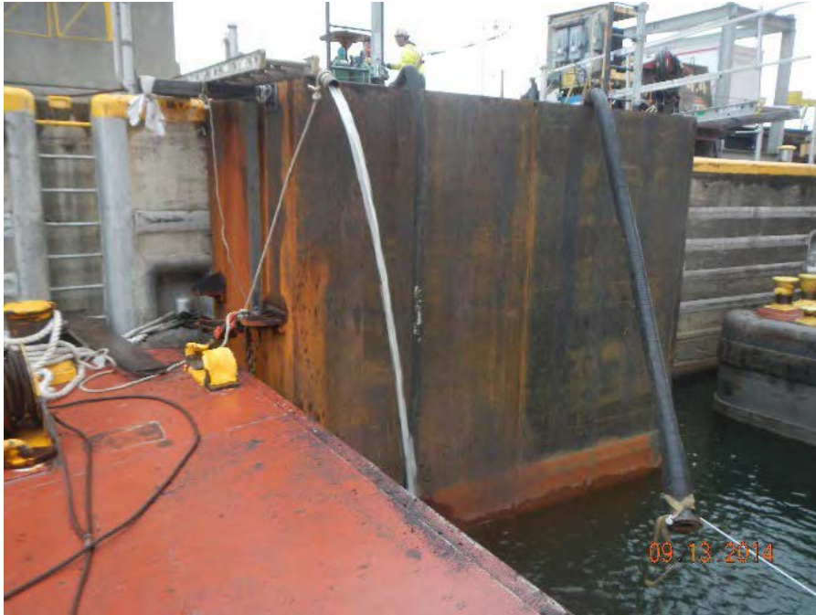
Figure 3. Example of an installed localized cofferdam.
