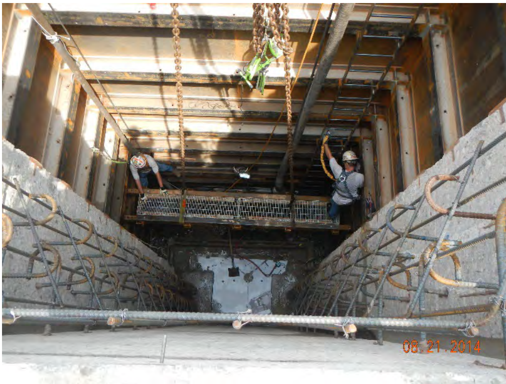
Figure 4. Example of the inside of a localized cofferdam.
