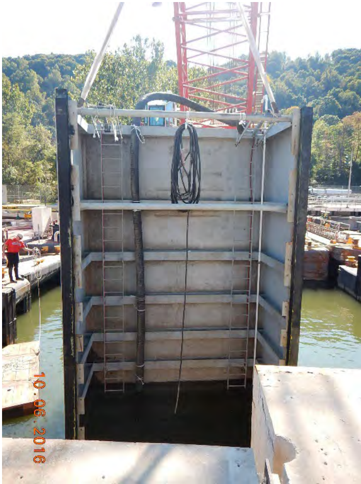
Figure 2. Localized cofferdam example.
