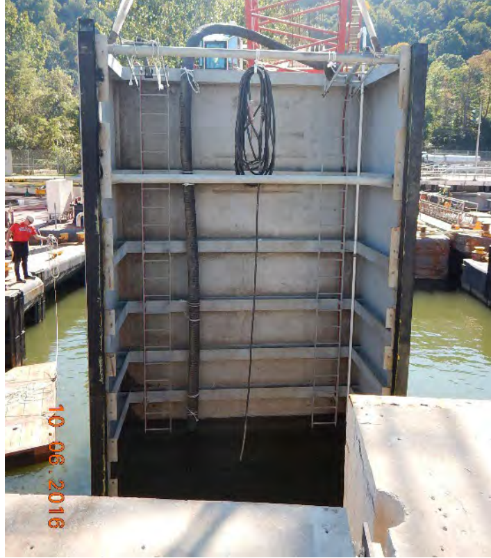
Figure 2. Localized cofferdam example.
