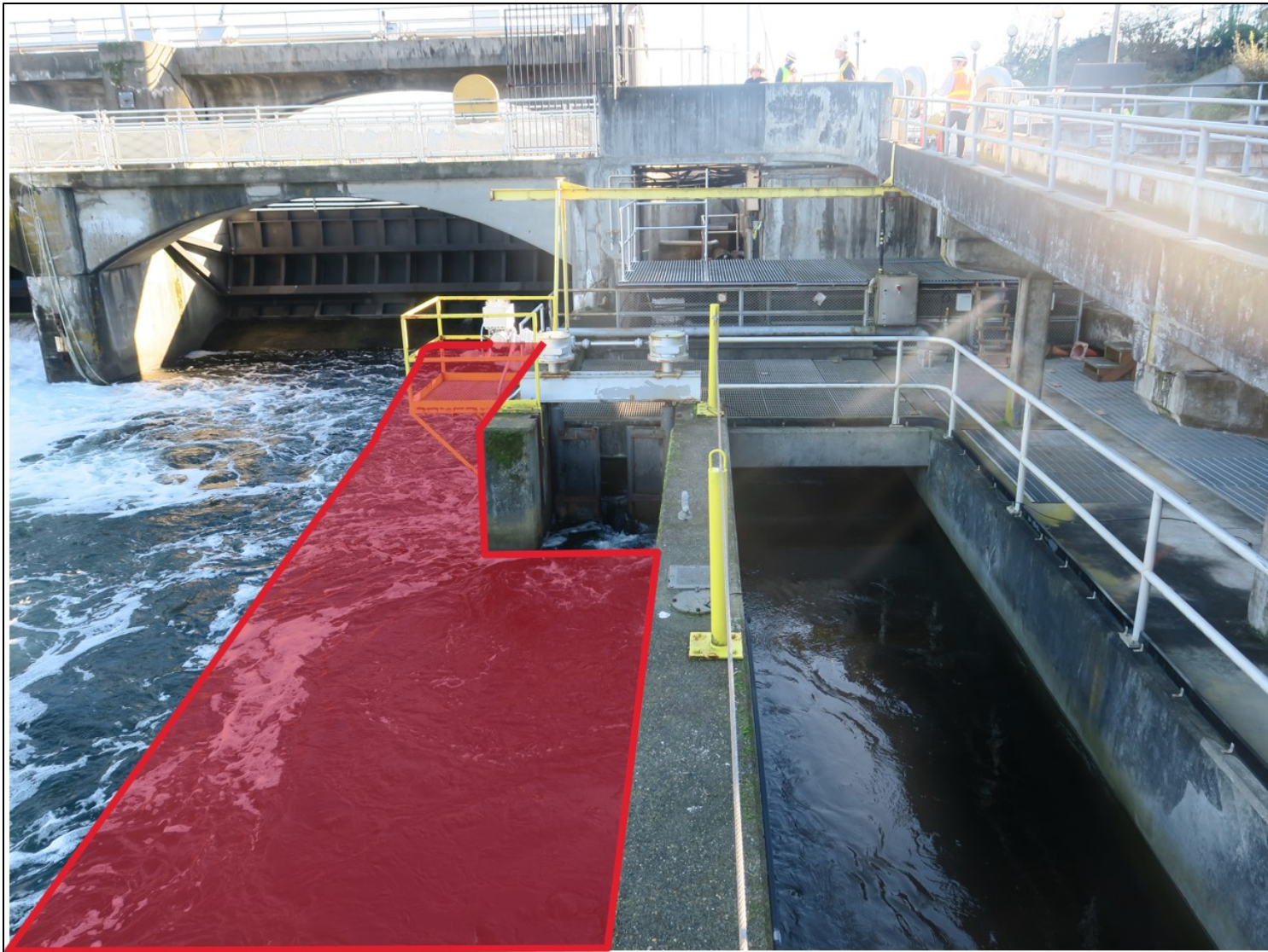
Figure 5. View of the scoured area (red box) between the stilling basin apron and the fish ladder from the observation platform.
