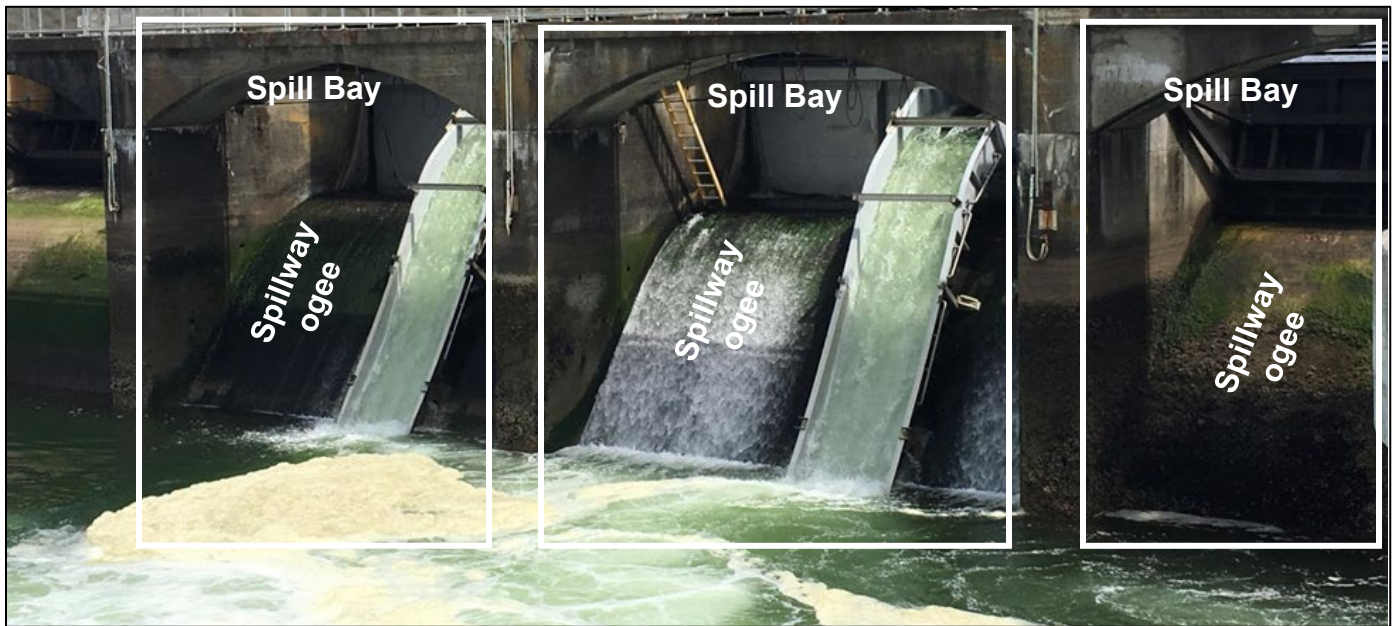
Figure 2. Location of the concrete stilling basin apron (top panel; outlined in white dashes) as seen in a 2016 bathymetric survey. The colors indicate depth with red as the shallowest and blue as the deepest. The bottom panel shows the configuration of three of the six spill bays and spillway ogees on the spillway. There are six spill bays at the Locks and each contains a spillway ogee. Note that the smolt flumes depicted in the lower figure are installed every spring to help provide juvenile fish safe passage to the Puget Sound and are removed prior to September, and so would not be present during the proposed repair operations.
