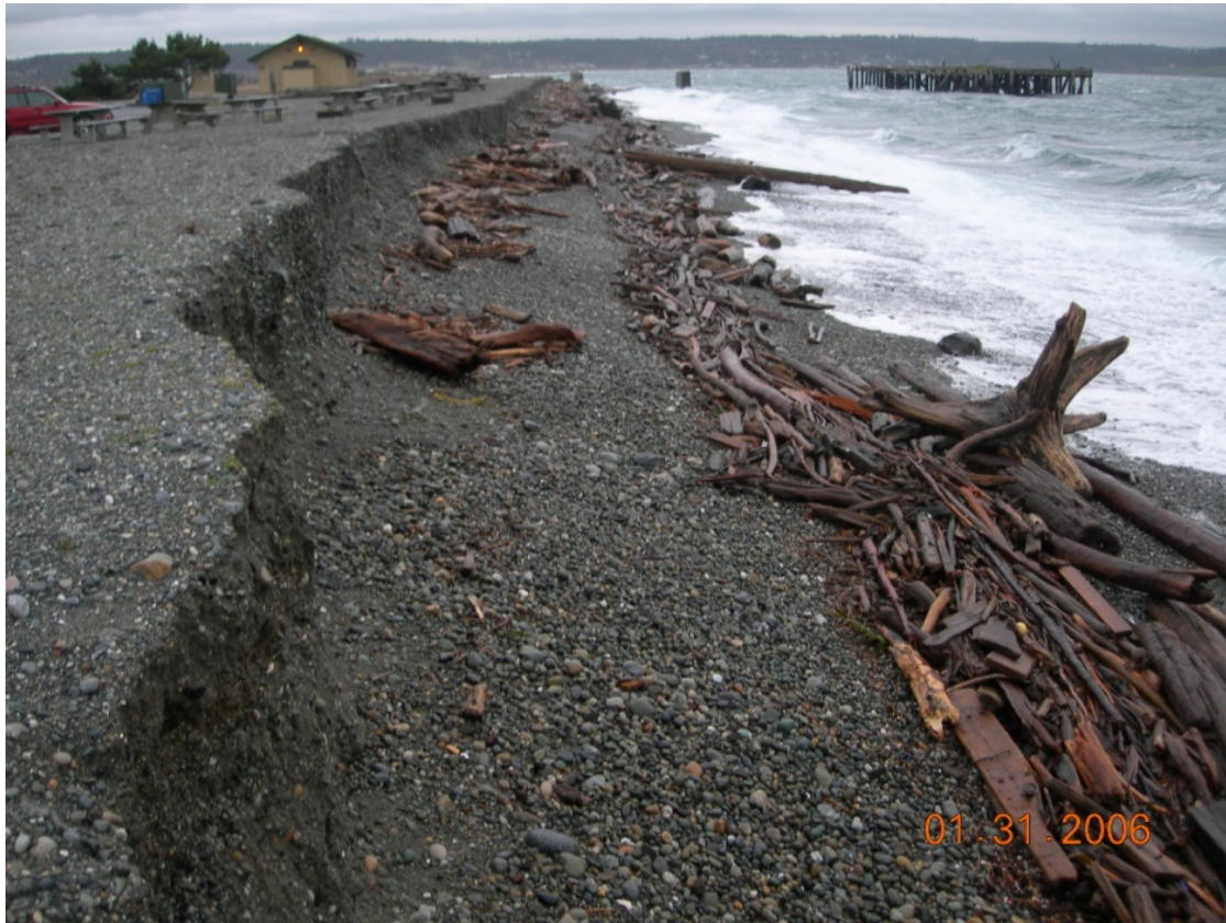
Figure 3. Shoreline erosion along the adjacent beach.
