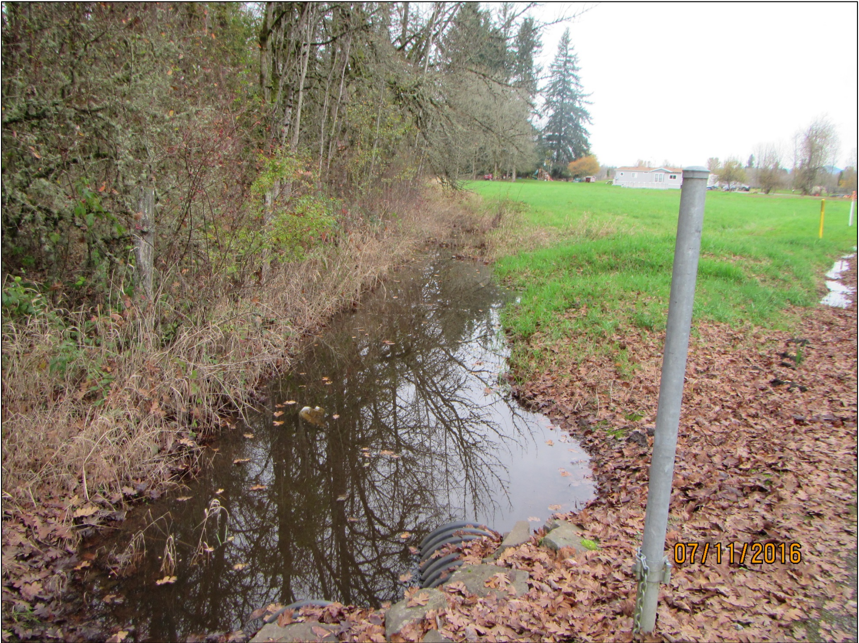
Photo 3: Looking westerly from offsite maintenance road outlet drainage channel from Wetland A and shotgun culverts.
